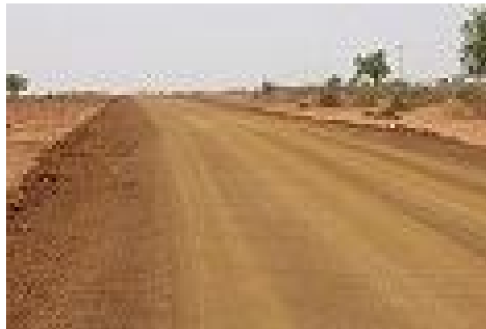
One of the roads under construction in the State
