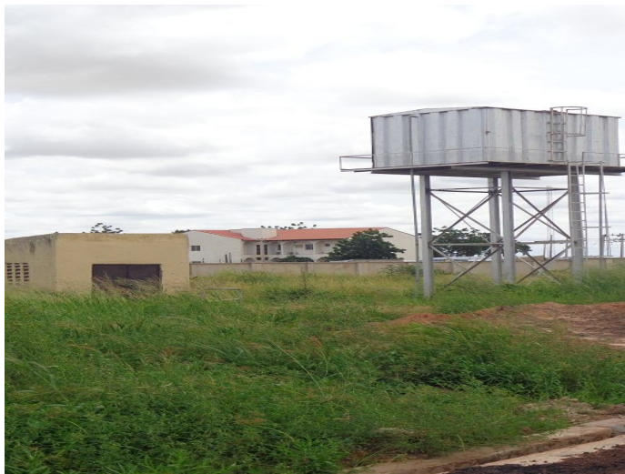
Functional Borehole to provide portable drinking water
