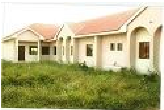
Newly constructed P.H.C. under the Geiidam's administration
