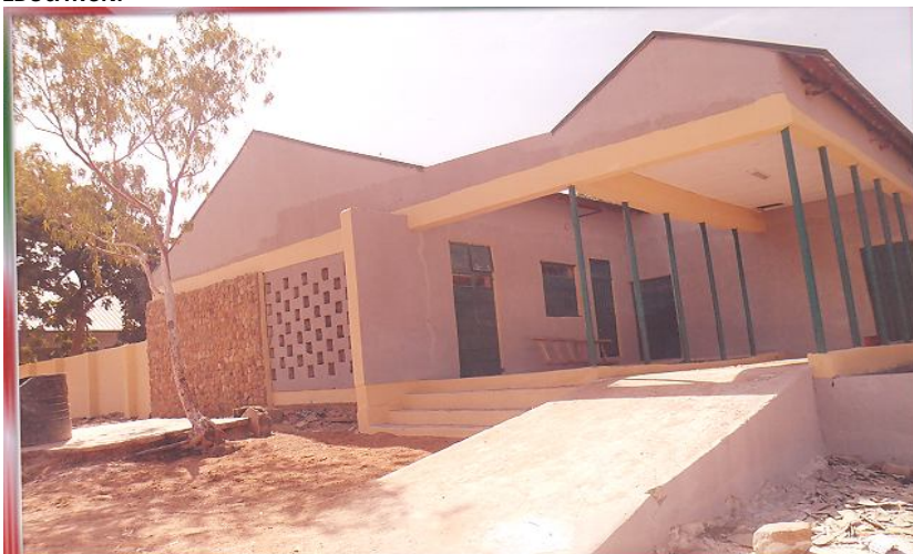
One of the renovated staff quarters
