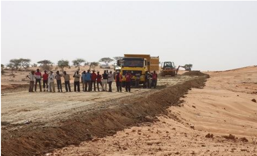
One of the road project under construction
