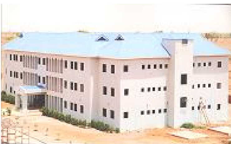
Administration Blocks at Turkish International College Mamudo HEALTH SECTOR
