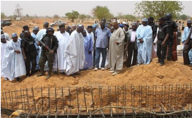
One of the drainages under construction being inspected by His Excellency Gov. Geidam
