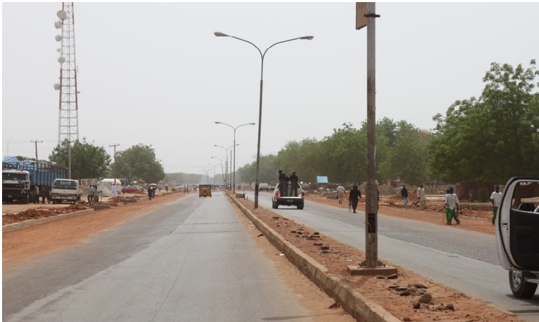
One of the Completed Township Road Project
