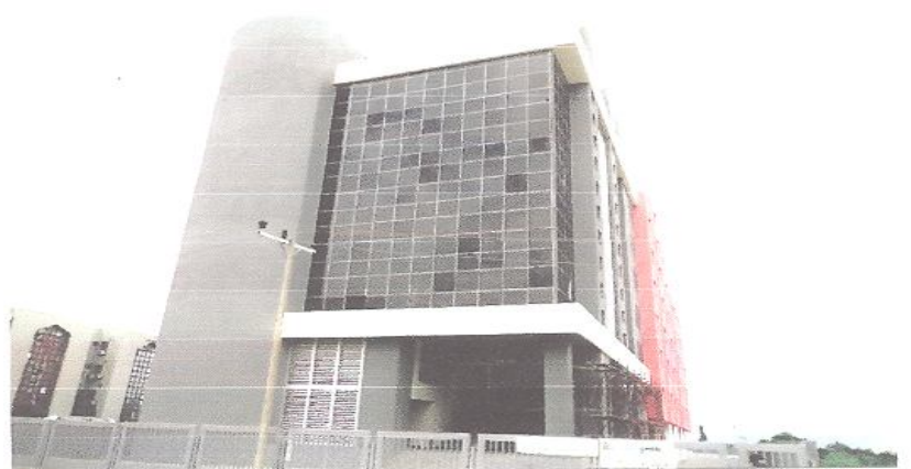
Investment House supervise by Min. of Housing under construction in Abuja
