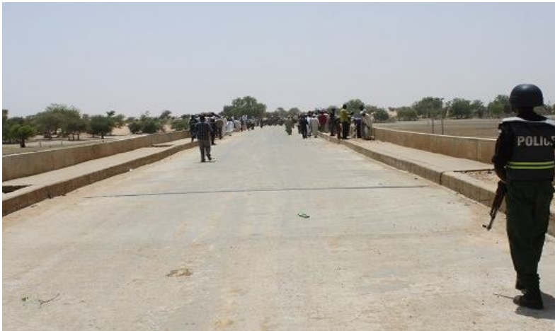
Potiskum-Jakusko bridges under construction
