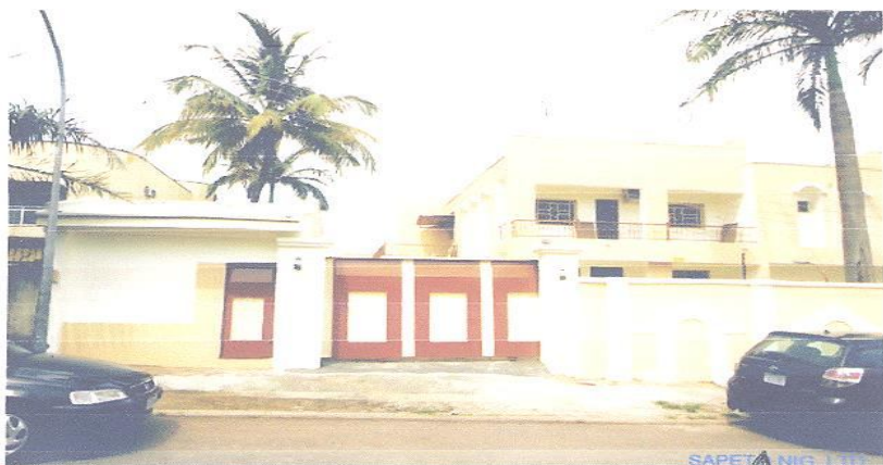
One of the renovated Staff quarters at Senior Secondary School
