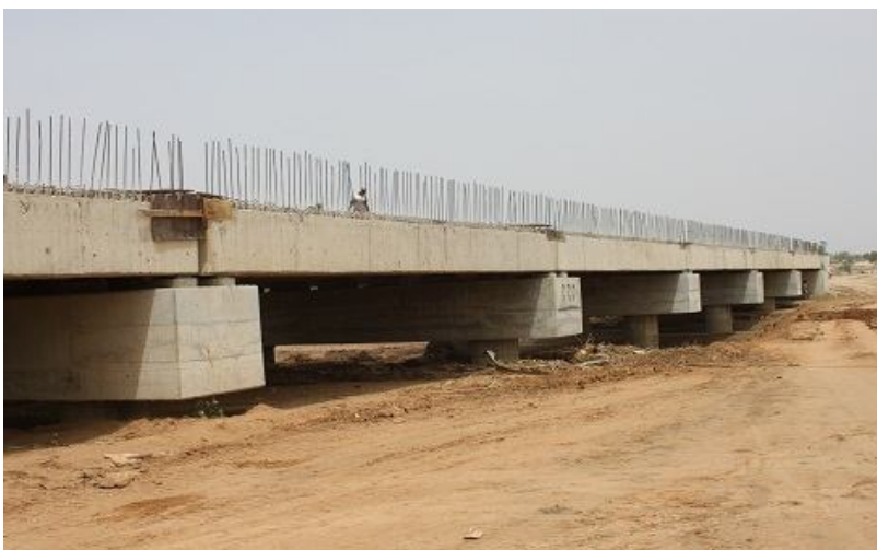
One of the bridges under construction
