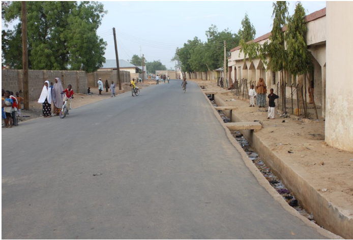
One of the estates roads projects completed
