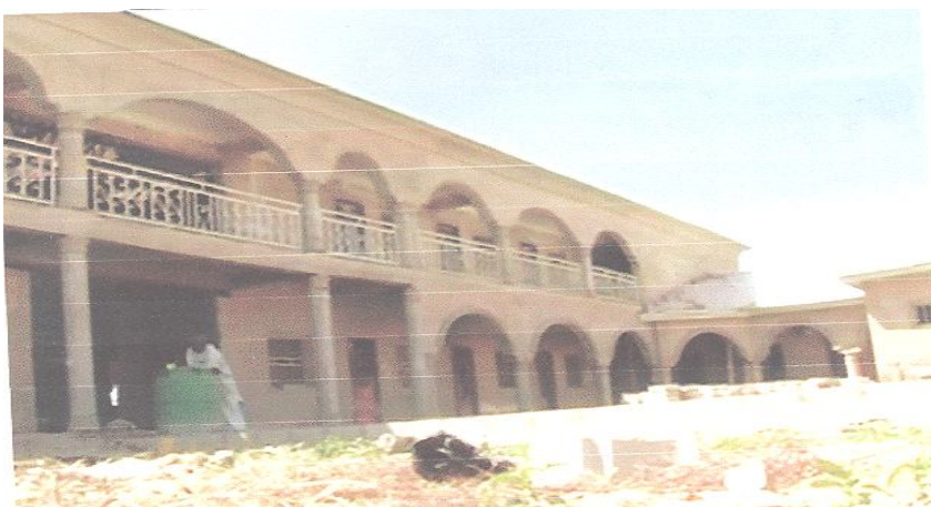
One of the Emir's palace under construction ON-GOING PROJECTS
