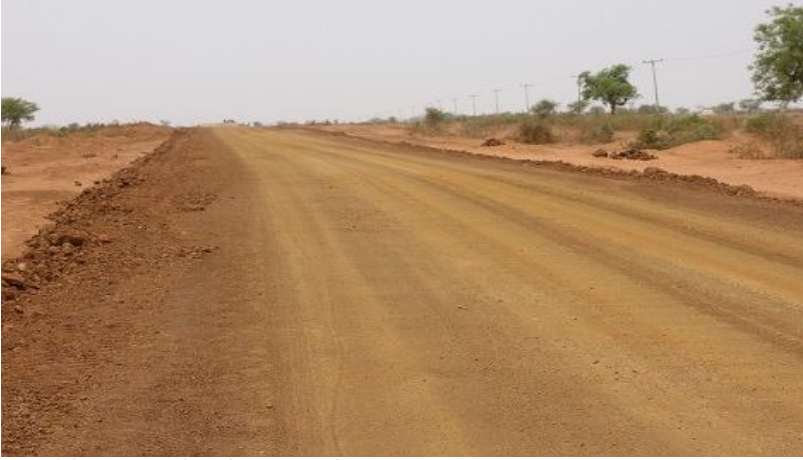
One of the State roads under construction
