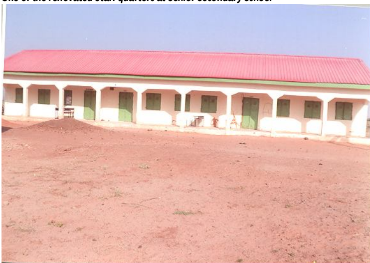
3 classrooms Block newly constructed in the year 2011
